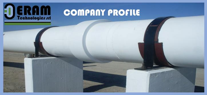
Pipeline Monolithic I/olation Joint
